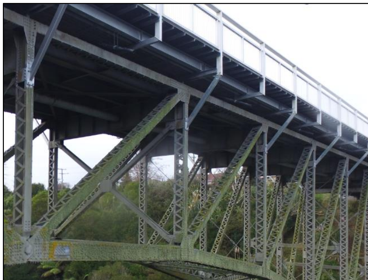
Figure A- 4: Drone photo showing lattice elements (2016).
