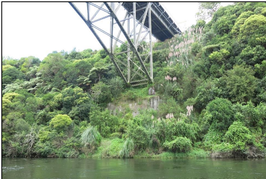
Figure B- 2: Southern bridge abutment slopes.
