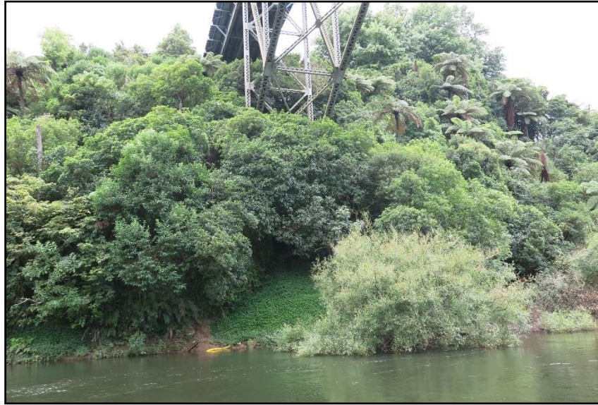
Figure B- 1: Northern bridge abutment slopes.
