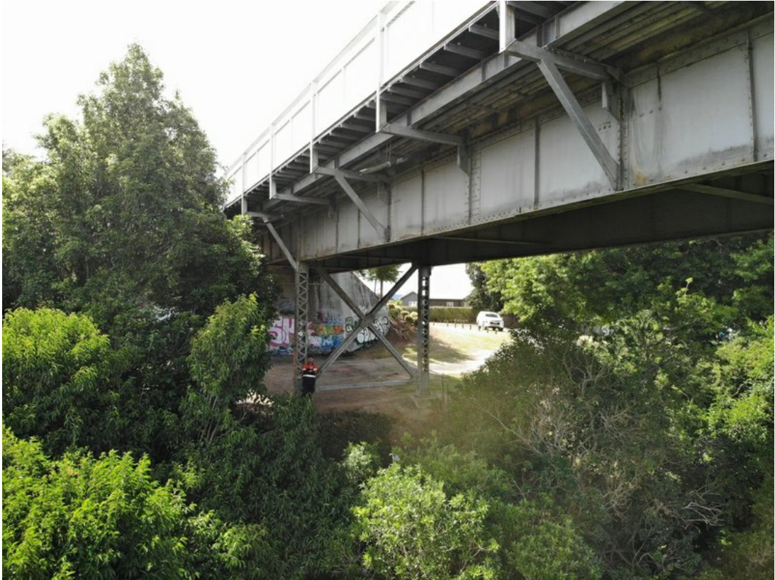
Primary Load Carrying Element (Element 1) : Steel beams on land spans generally in good condition. View from D/S side looking towards Cambridge end.
