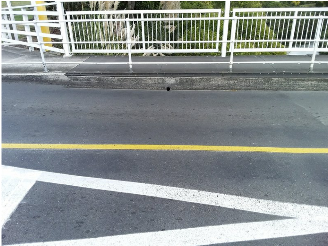
Superstructure Drainage (Element 15): Clear drain hole on kerb.
