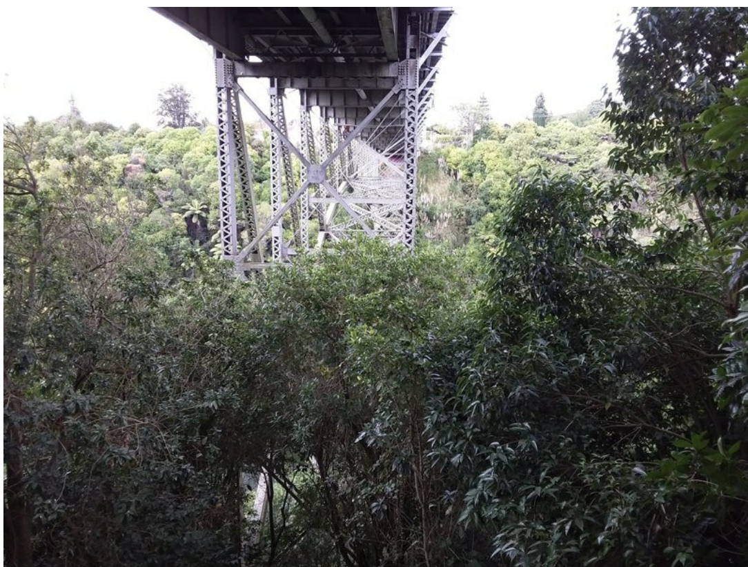
Invert / River Bed (Element 25): Could not access due to steep banks and dense vegetation.
