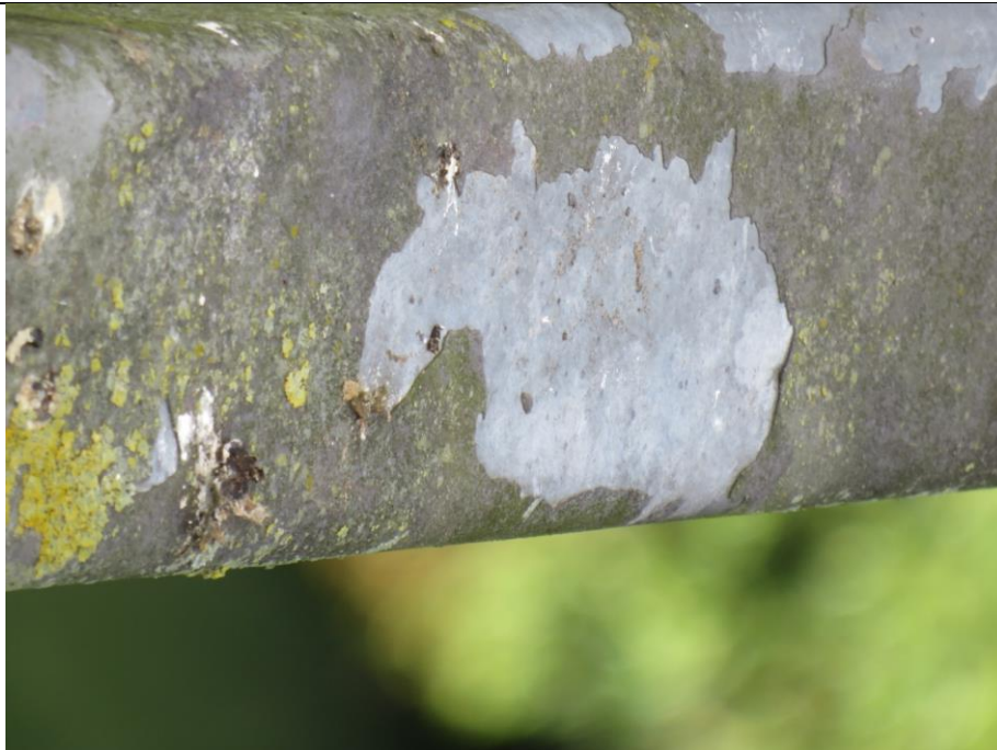
COATING DELAMINATION
