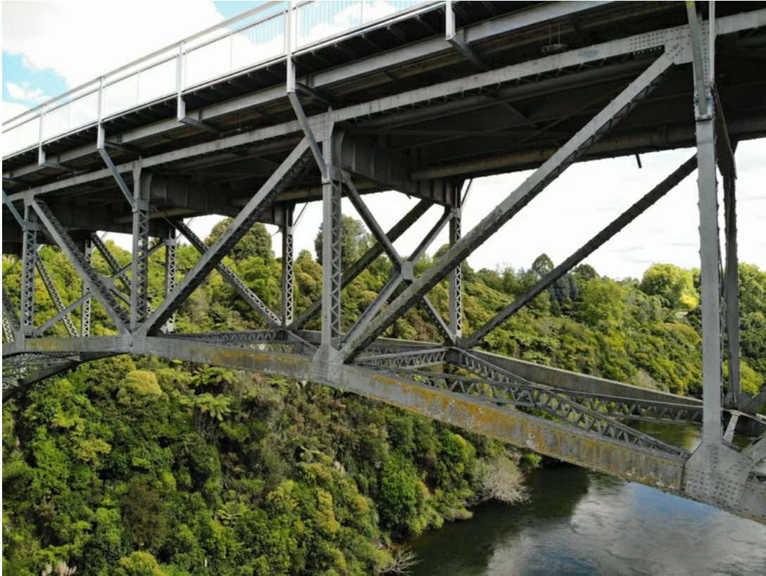
Painting: Superstructure Elements (Element 18): The general condition of the entire coating system is considered stable. View from U/S side.
