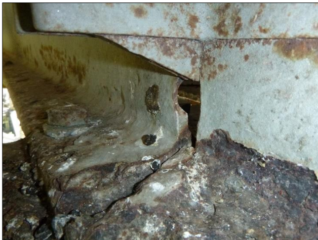
Figure 4-13 - Web may be deformed investigate during painting at T10.
