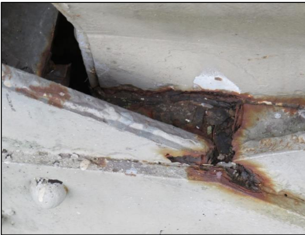
Figure 4-14 - Pitting and crevice corrosion at central pin
