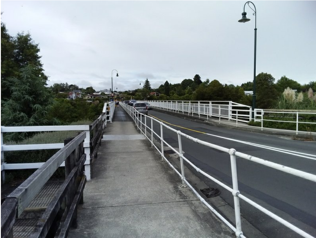
View Along Carriageway (increasing direction)
