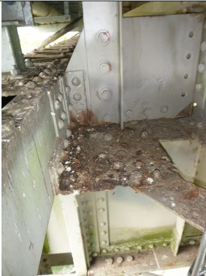
CROSS BRACE AND TRANSOM CONNECTION
