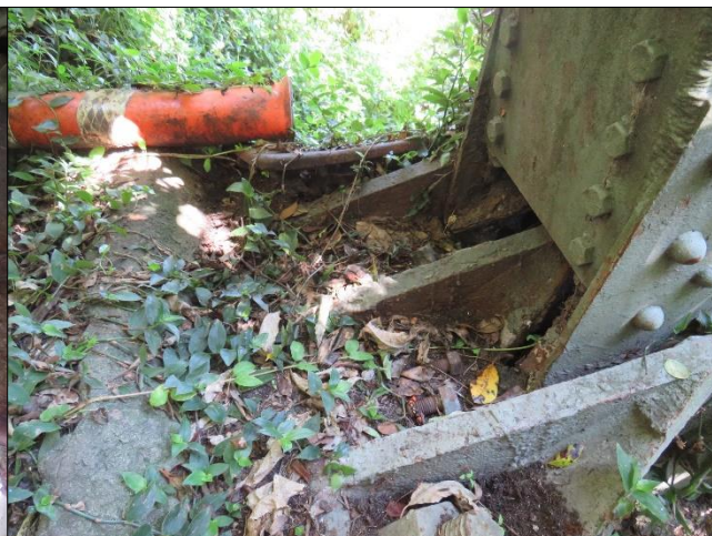
Figure 4-17 - Vegetation build-up at ground level Pins
