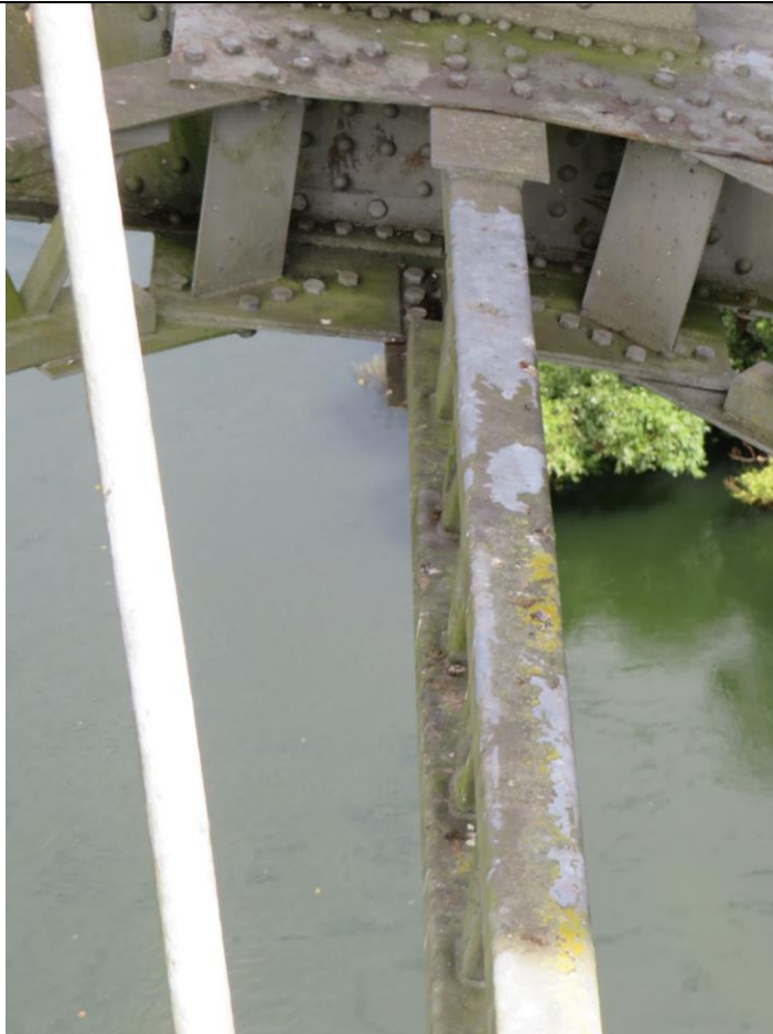
COATING DELAMINATION
