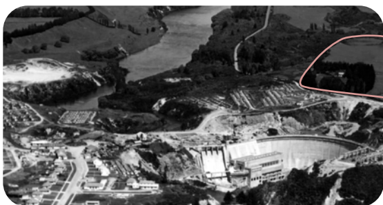
Construction of Karāpiro Dam c1940's showing indicative outline of future Karāpiro Lake Domain. Photo credit: Unknown
