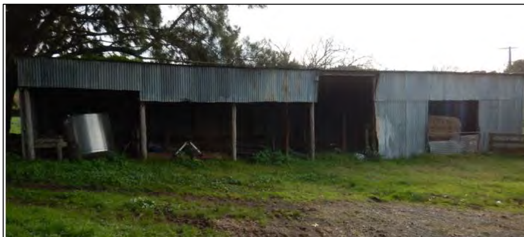
Figure 20. Photograph showing the corrugated iron shed, looking west
