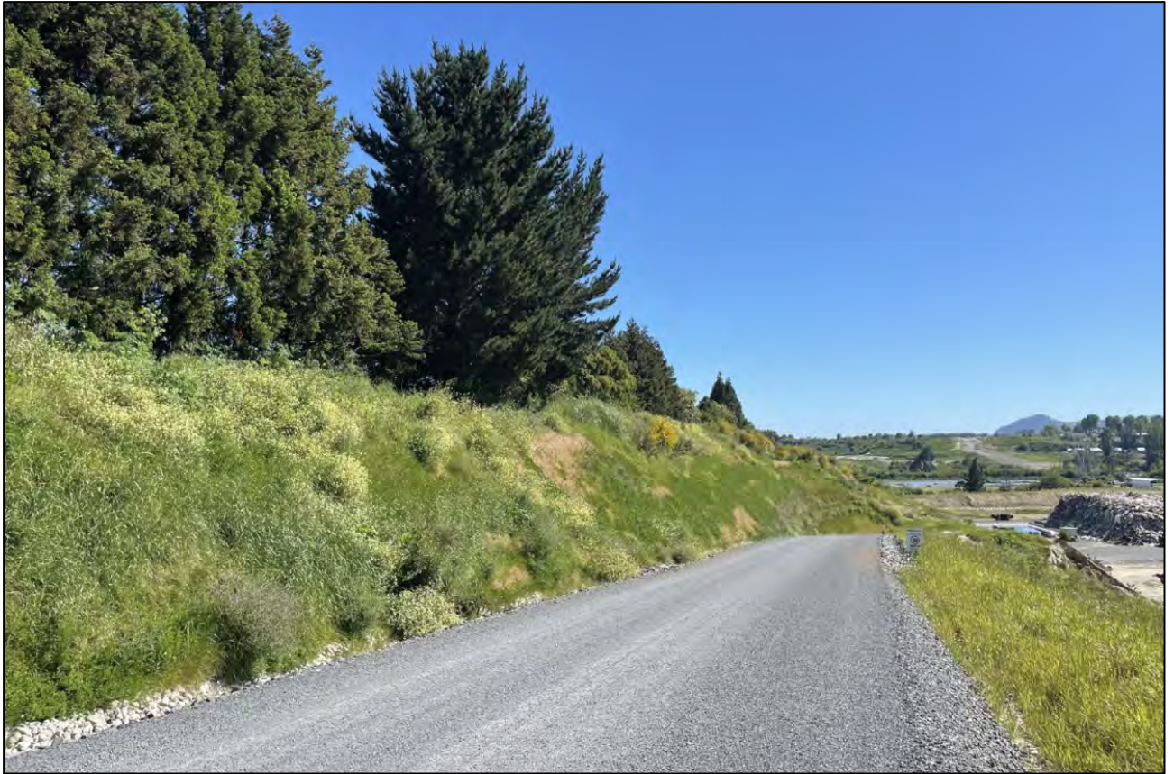
Figure 27: Site visit photo showing the internal access road along the western boundary of the site towards the waste recycling operation (facing north).
