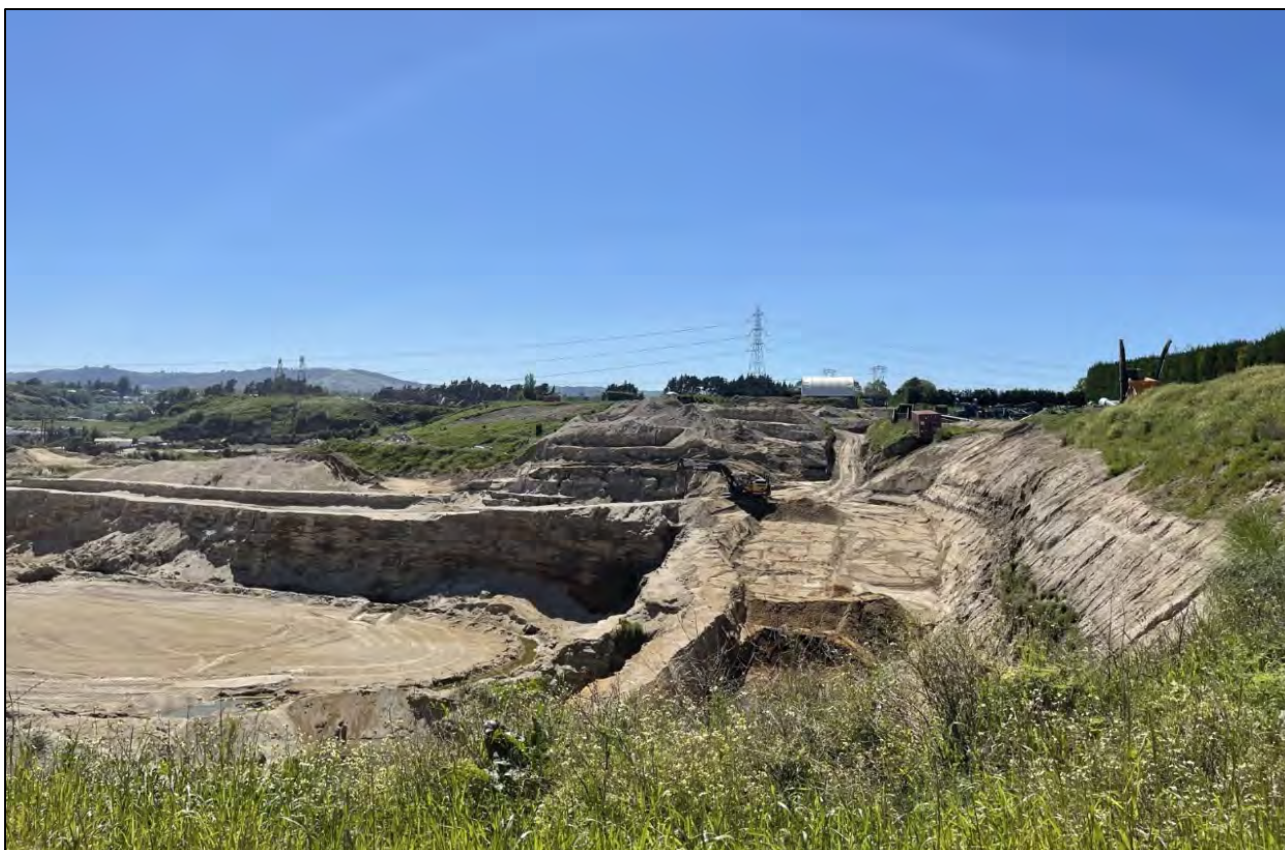
Figure 23: Site visit photo showing the quarry area within proposed Stage 1 (facing east).
