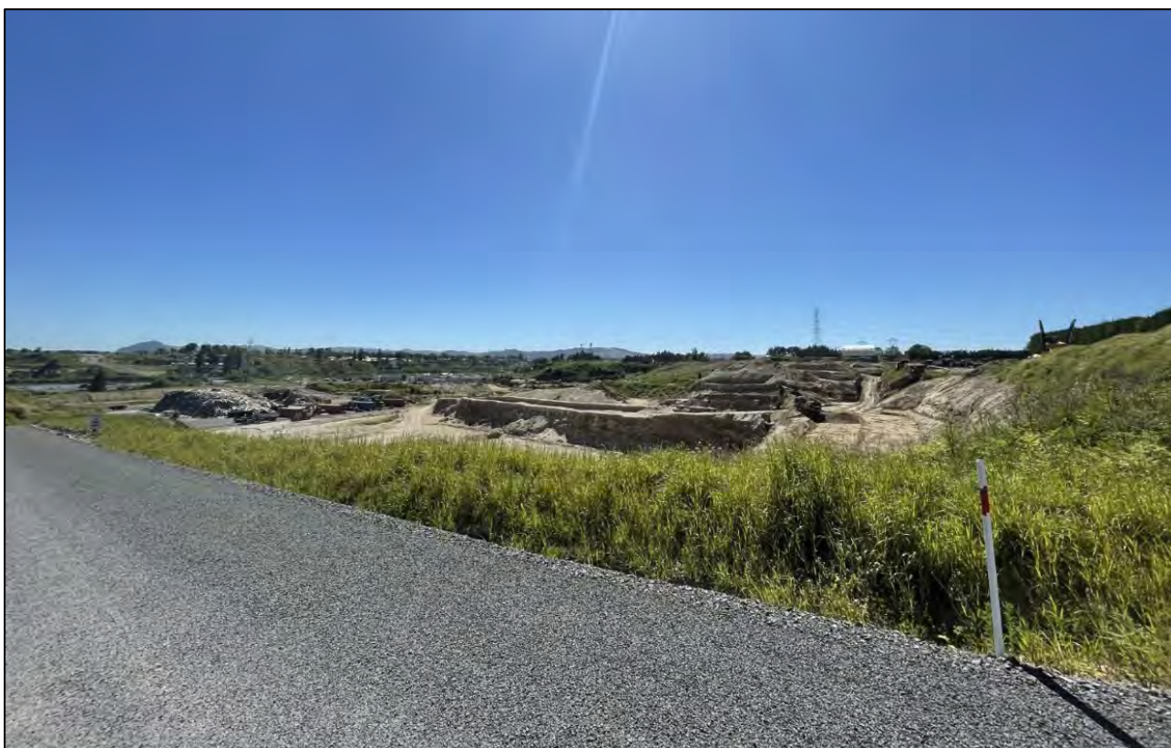
Figure 22: Site visit photo showing the quarry from the western boundary of the site (facing northeast).
