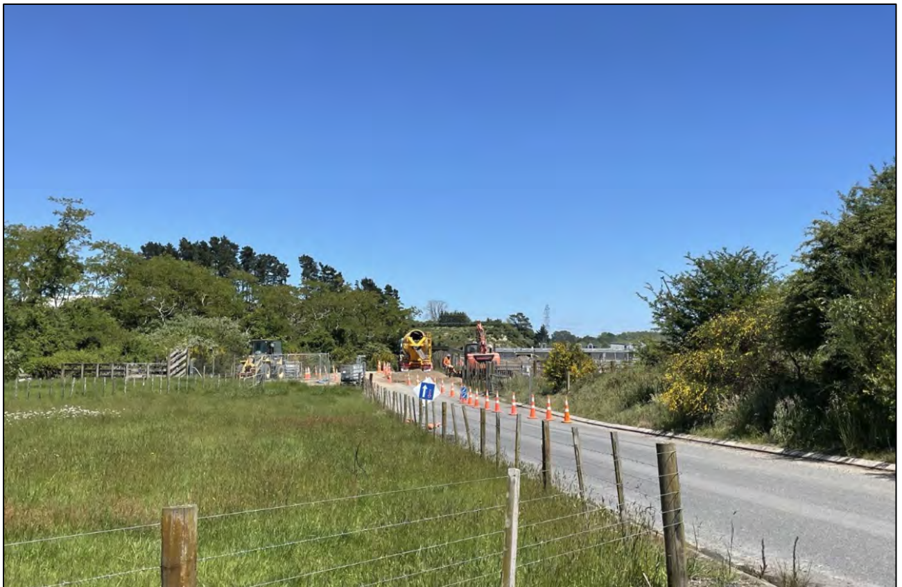
Figure 36: Site visit photo showing the view towards the site from the WWTP entrance (facing southwest).
