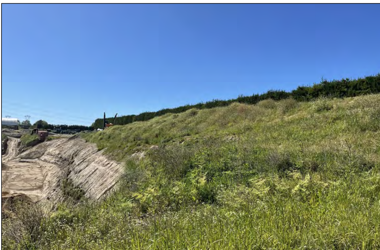
Figure 24: Site visit photo showing towards the southern boundary of the site marked by the pine trees and showing the ground level where the site will be raised to (facing east).
