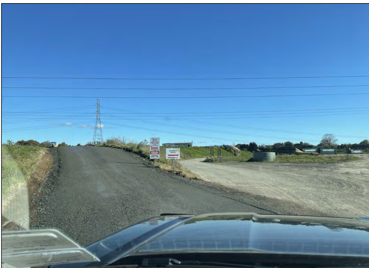
Figure 14: Site visit photo showing the accessway (starting to be sealed) along the southeastern boundary (facing southwest).
