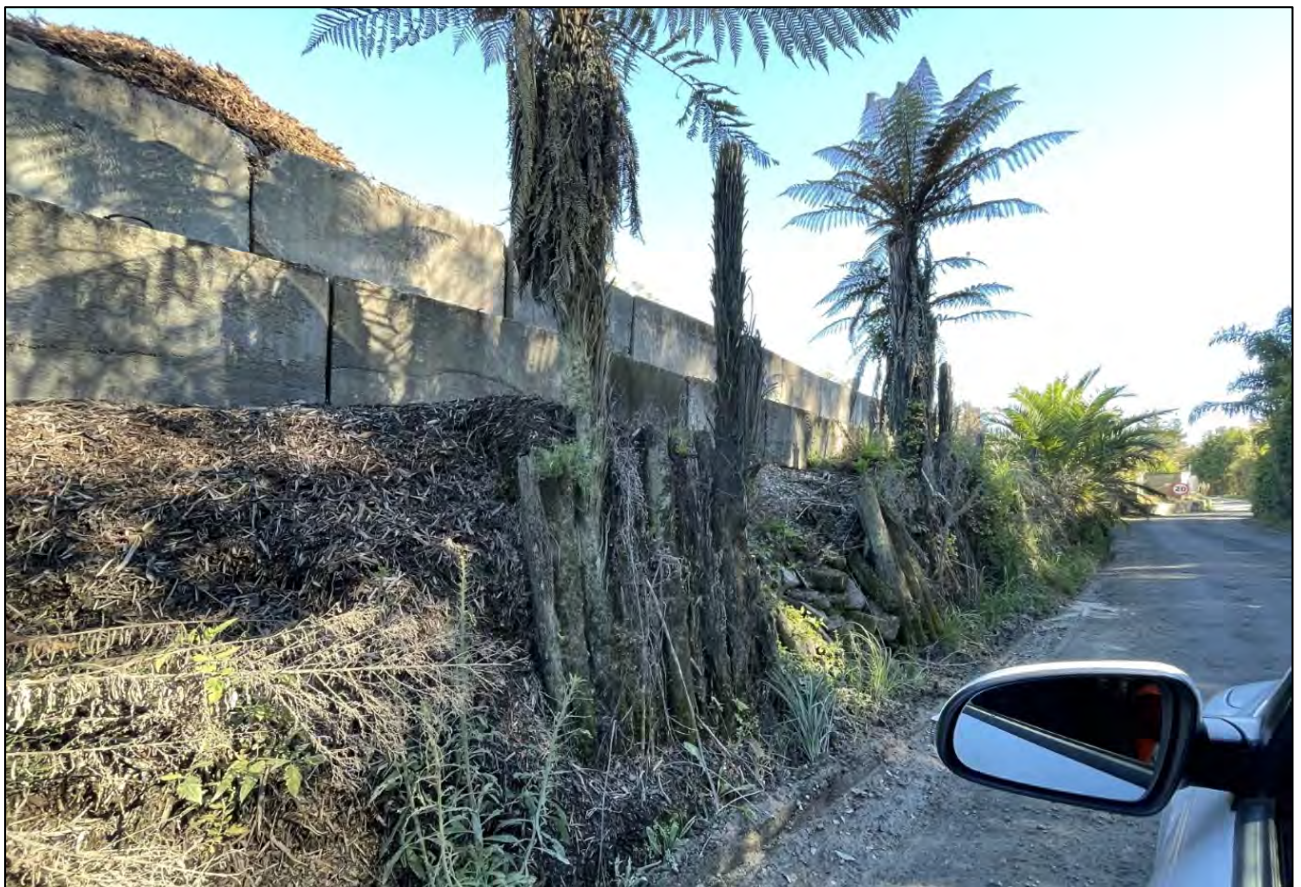
Figure 12: Site visit photo showing the accessway with retaining next to the landscaping business.
