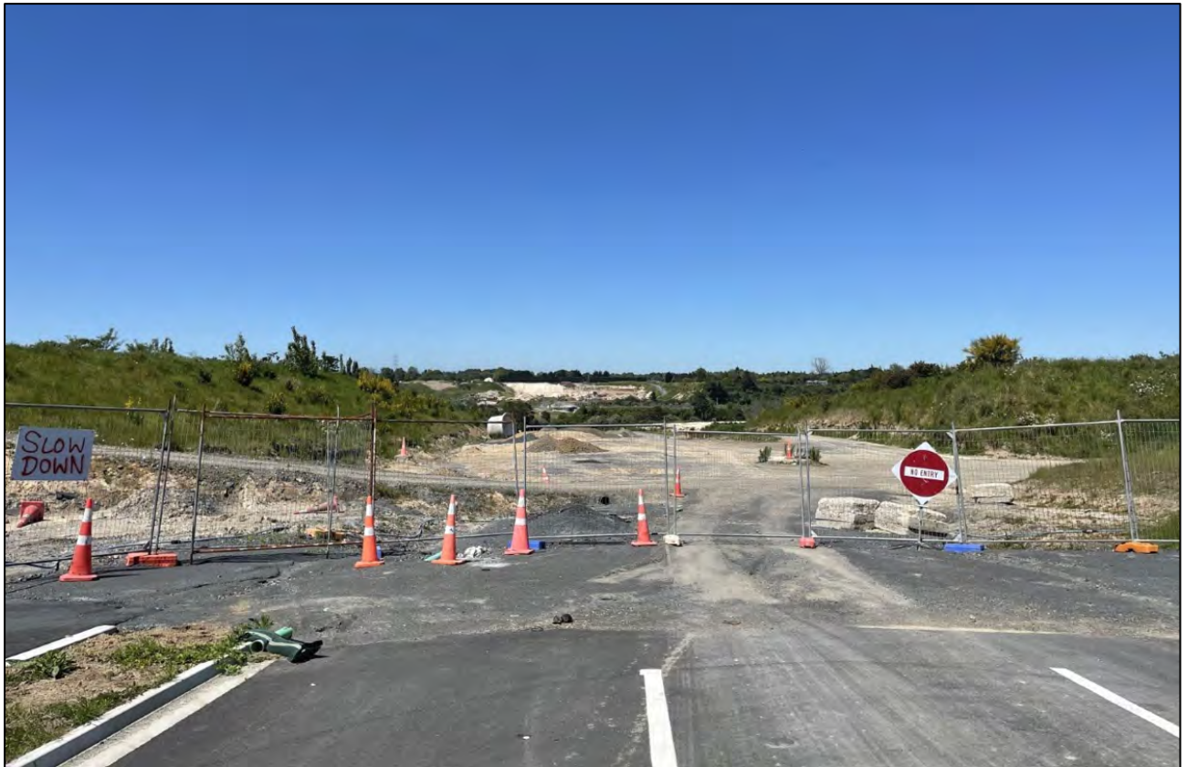
Figure 35: Site visit photo showing the view of the site from the southern exit off the new Cambridge Road roundabout (facing south).
