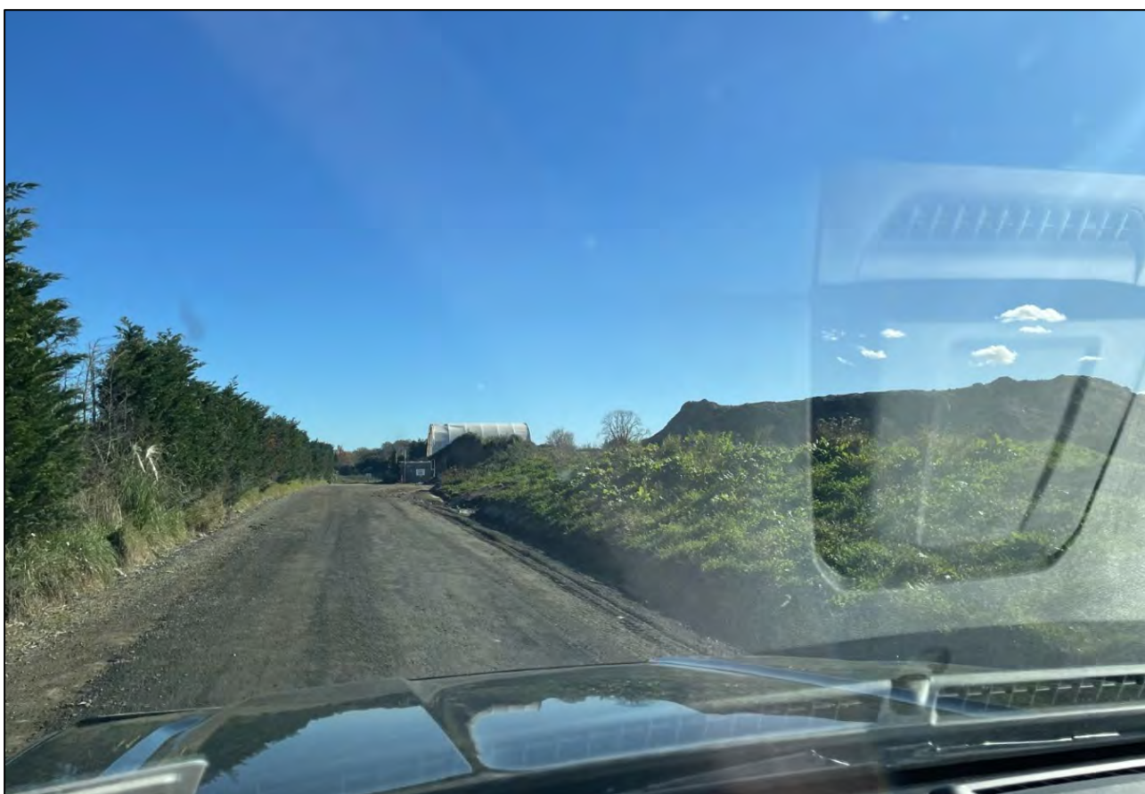
Figure 16: Site visit showing the haul road, pine trees and ground level along the southern boundary (facing west).
