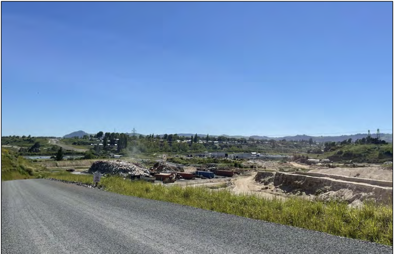
Figure 28: Site visit photo showing the waste recycling operation from the western boundary of the site (facing north).
