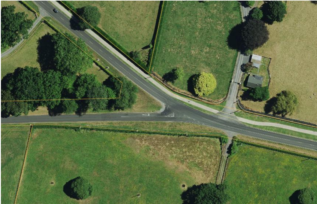
Figure 7-6: Existing Maungatautari Road/Lamb Street Intersection (Source: WDC Maps)
